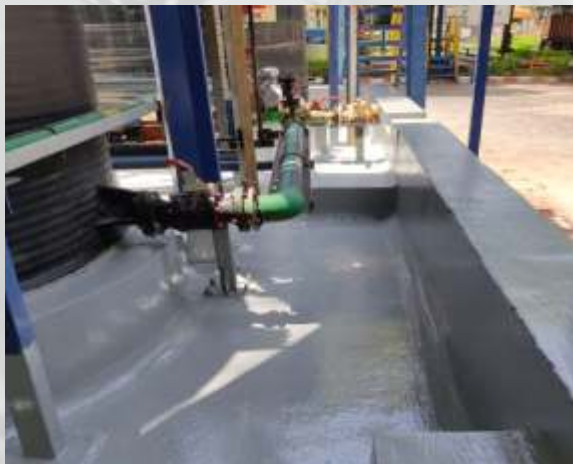
Chemical Resistance coating on dyke area, chemical production area, RO/DM plant
